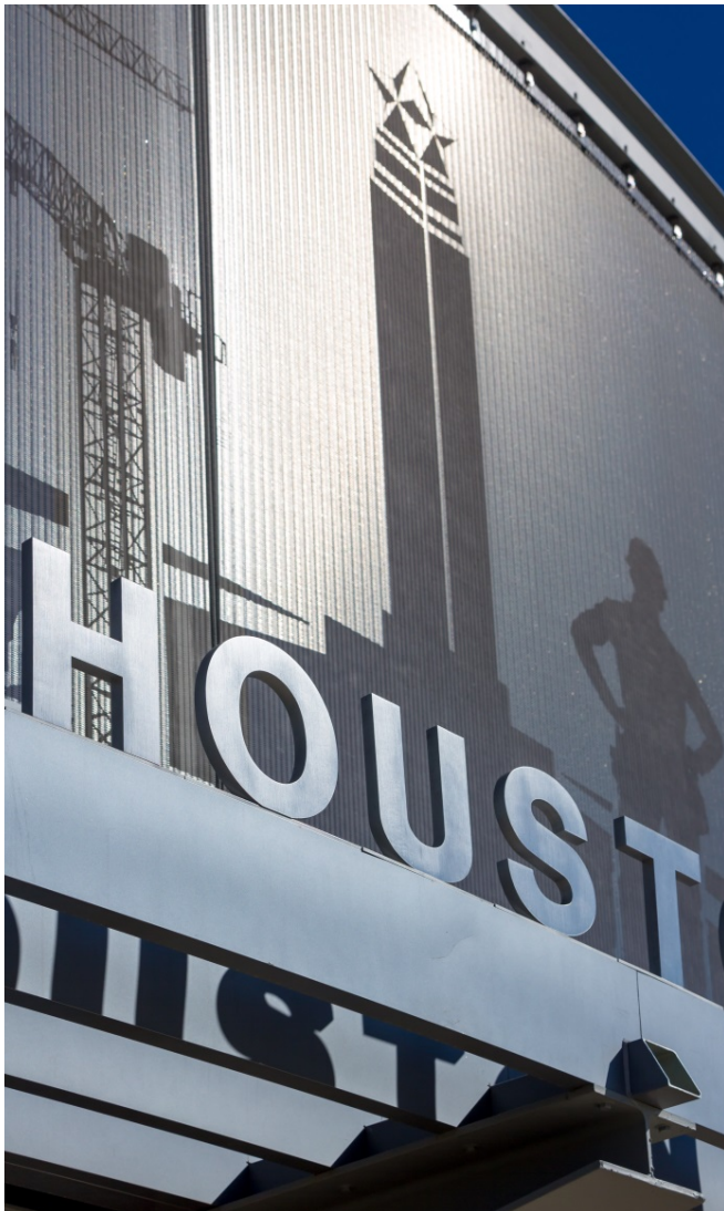
Picture 4: Using a special etching process developed in-house, GKD created a silhouette-like panoramic view on the balustrade.
