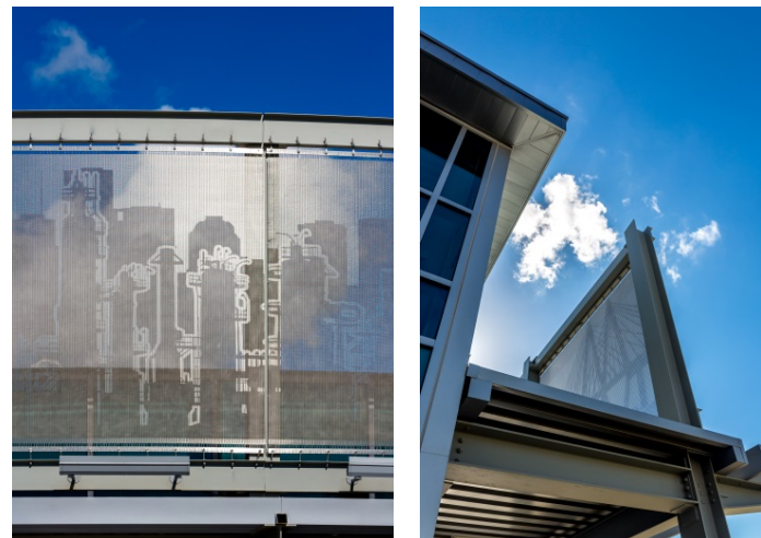
Picture 6-7: Through etching, the complexity of the motif had to be embedded in multiple levels to lend the images the desired spatial depth.
