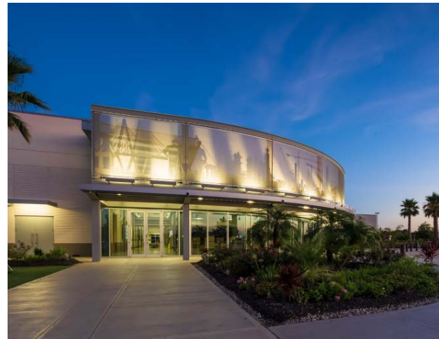
Picture 3: At night, spotlights lend the applied motifs by GKD the appearance of a shadow theater using targeted light accents.
