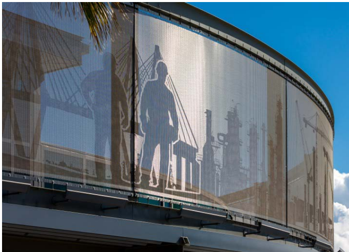
Picture 2: GKD-USA used a new etching technique for the design of the 100 square meter roof parapet, which is made from semi-transparent Omega 1510 stainless steel mesh.
